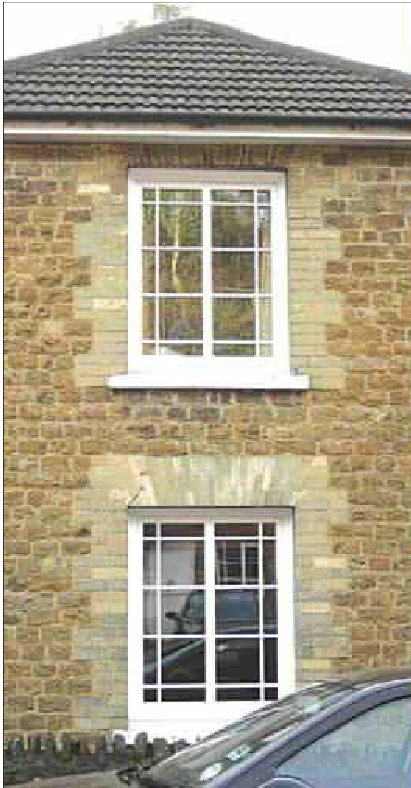
Replacement windows in a Bargate stone cottage.
