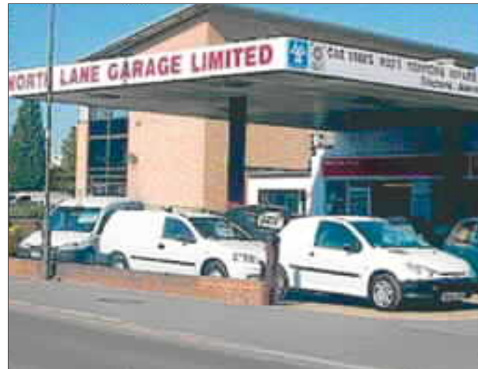
North Lane Garage has been refurbished.
