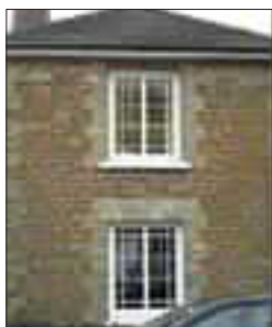
The replacement windows in this Bargate stone cottage are in keeping with the style.
